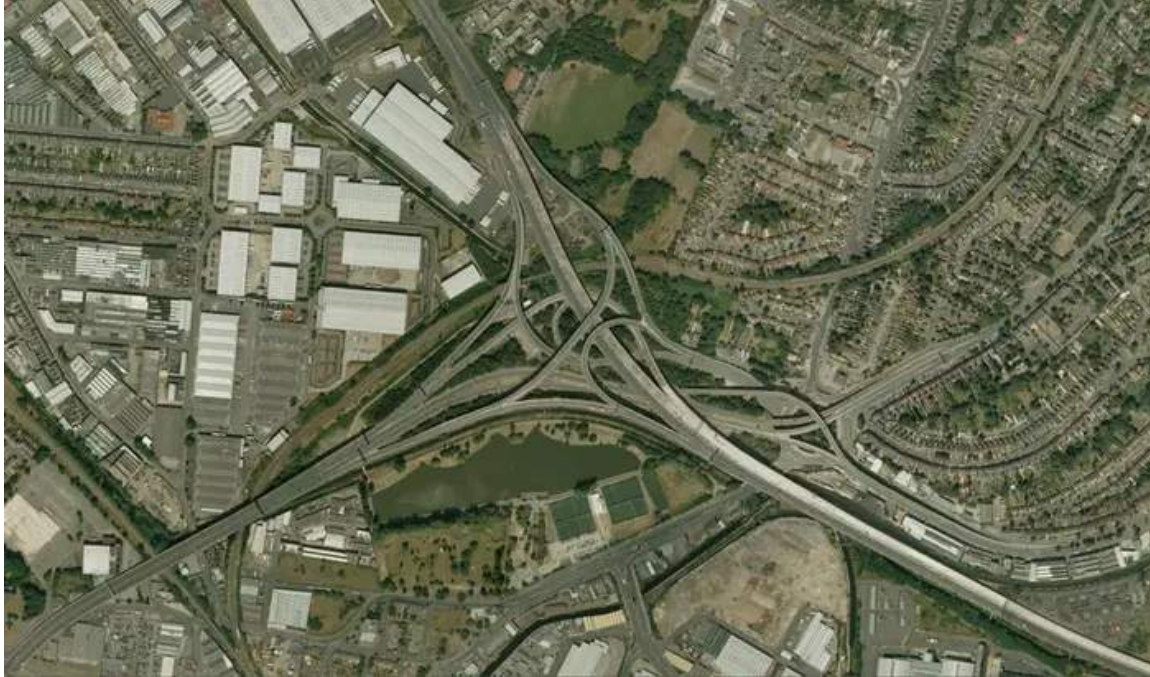
Satellite photo of Birmingham's Spaghetti Junction
