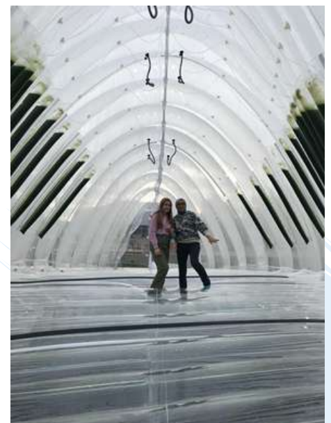
This structure used the carbon dioxide we were respiring to stay inflated
